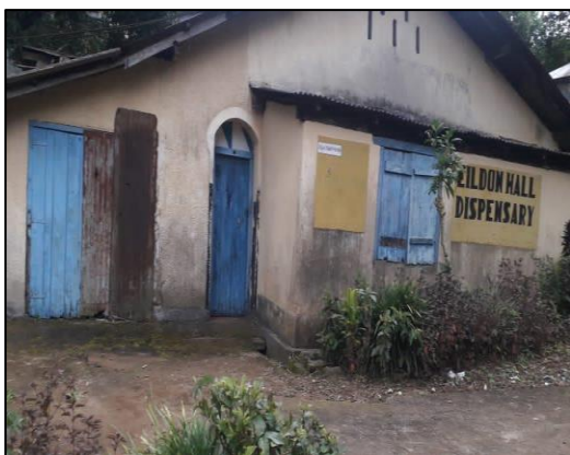
Figure 5: Eildon Hall Dispensary
